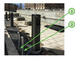
If optional, the integrated 1Base crash protections are a part of the installation. These shall be installed so the pervading screws (1) of the bollards are just above ground level. This to ensure easy switch of damaged poles (2) in case of any vehicle crashing into it. 1Base has pre-drilled holes used as attachement points for the crash protection(3).
