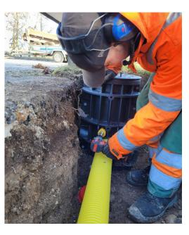
The foundation should be placed in a cavity large enough to accommodate the excavated ground materials, which can be compacted both underneath and on the sides of the foundation. Ensuring the materials are thoroughly packed to fill the
